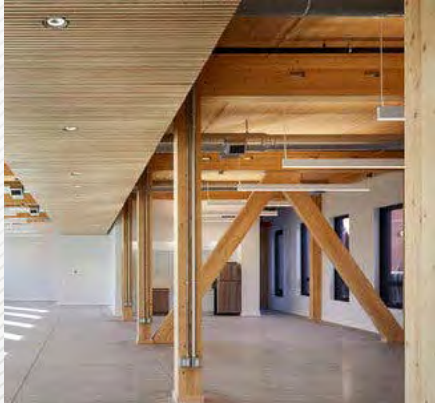
320 Wythe Avenue in Williamsburg — an example of mass timber design.
